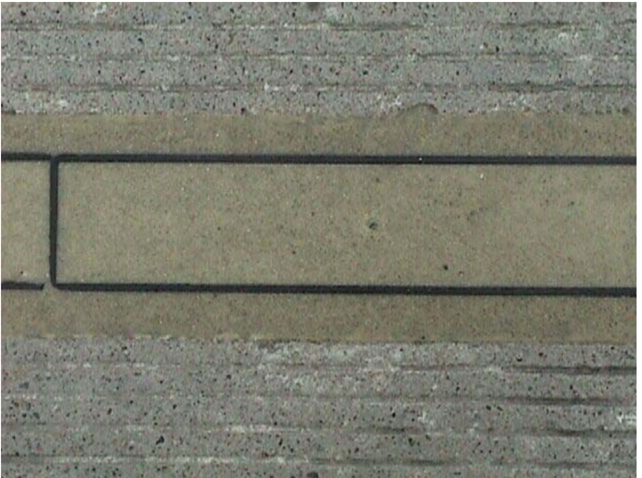
Figure 1 Quartz Sensor Installed in Roadway
